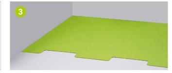
**3.** The sheets can be cut to size using a carpet knife. A gap of 10 mm must be left between the edge of the underlay and the walls/ openings. When installing the GREEN LIGNIN "puzzle"-format, we recommend cutting a straight edge to the walls.
